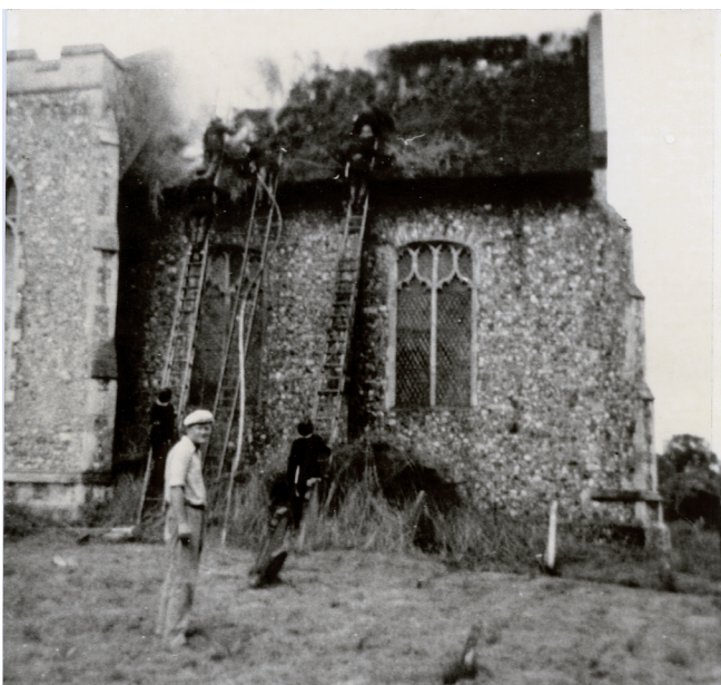
In 1963 the thatched chancel roof on St Helen’s church caught fire. Malcolm Davey looks back to the camera in despair as firefighters are seen tackling the blaze and removing the reed.
